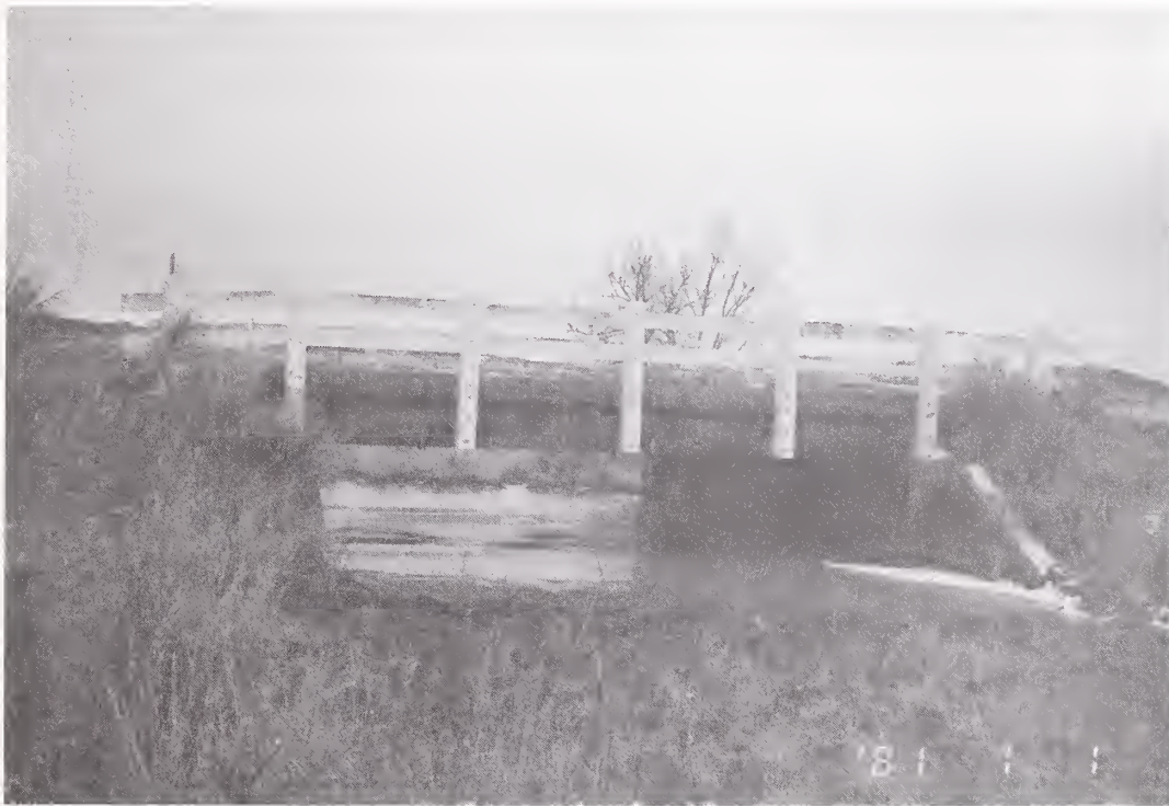
Cottonwood Creek Bridge. The bridge is typical of timber bridges built in the rural areas of Montana during the 1920s and 1930s.
